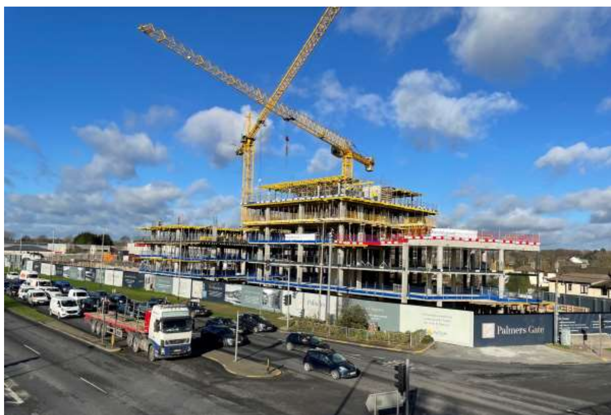
Fig. 1 – Palmerstown Strategic Housing Development Under Construction (Feb, 2022)
