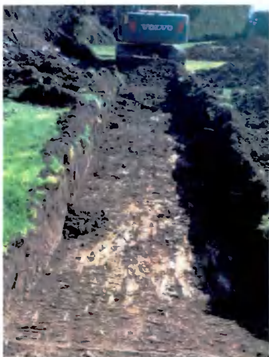
Fig. 14. Trench 4, looking southeast.
