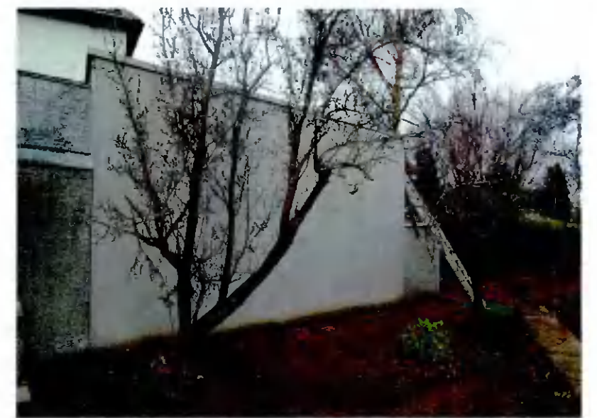
View, from adjoining garden of an extension built at 100 Barton Drive, showing precedent for which planning permission was granted.
