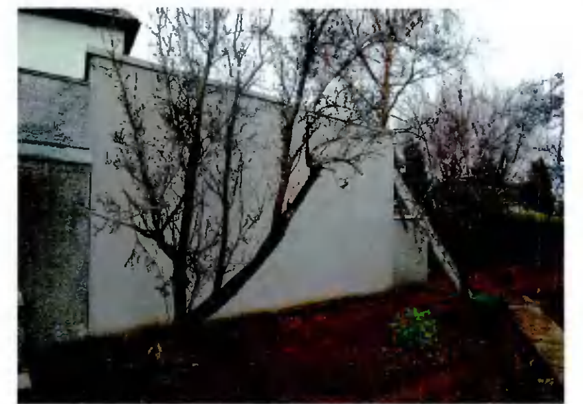
View, from adjoining garden of an extension built at 100 Barton Drive, showing precedent for which planning permission was granted.
