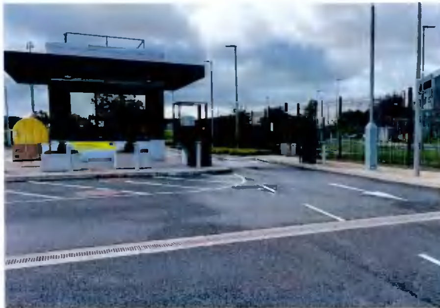
PHOTO No.03 SINGLE EXIT LANE. HEAVY DUTY TRAFFIC BARRIER TO BE REMOVED AND PROPOSED NEW TRAFFIC ARM IN NEW POSITION.
