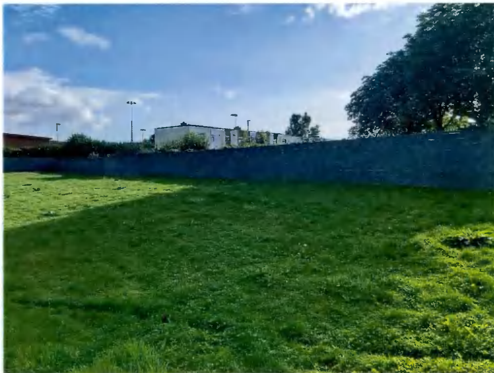
Plate 2: Cement block eastern boundary wall, facing northeast
