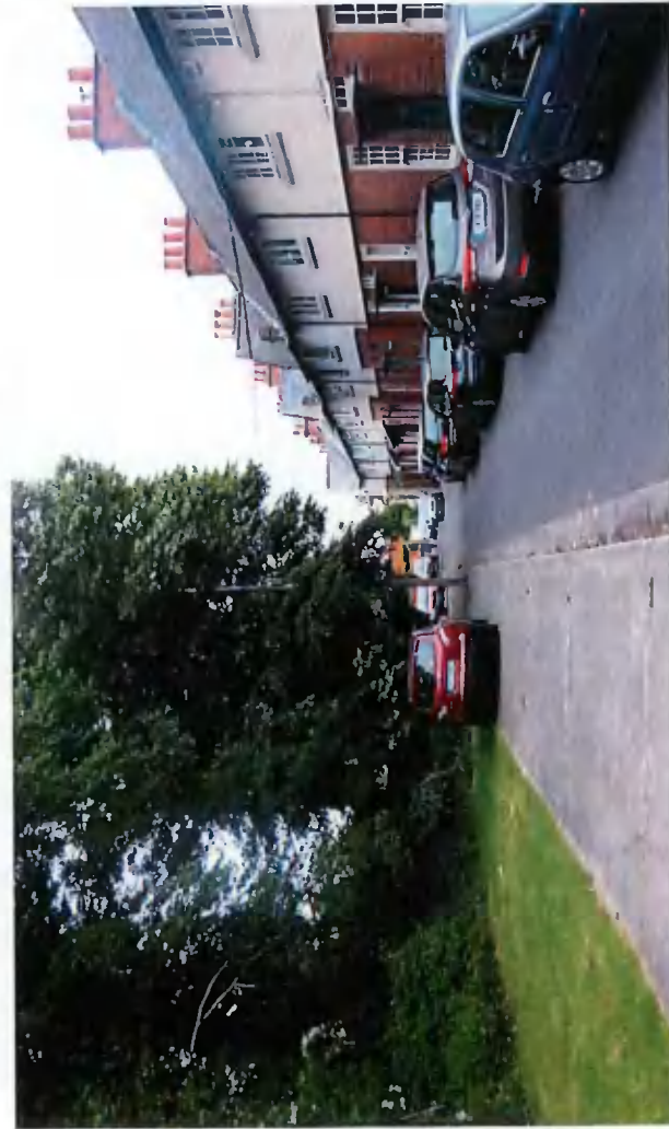
Fig. 19 – View north on St. Patrick's Cottages (ACA) with Mill House site on left
