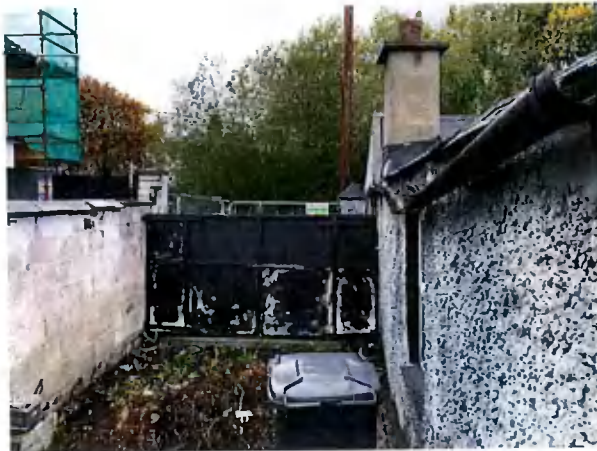
Figure 34 – Existing cottage garden gate access.
