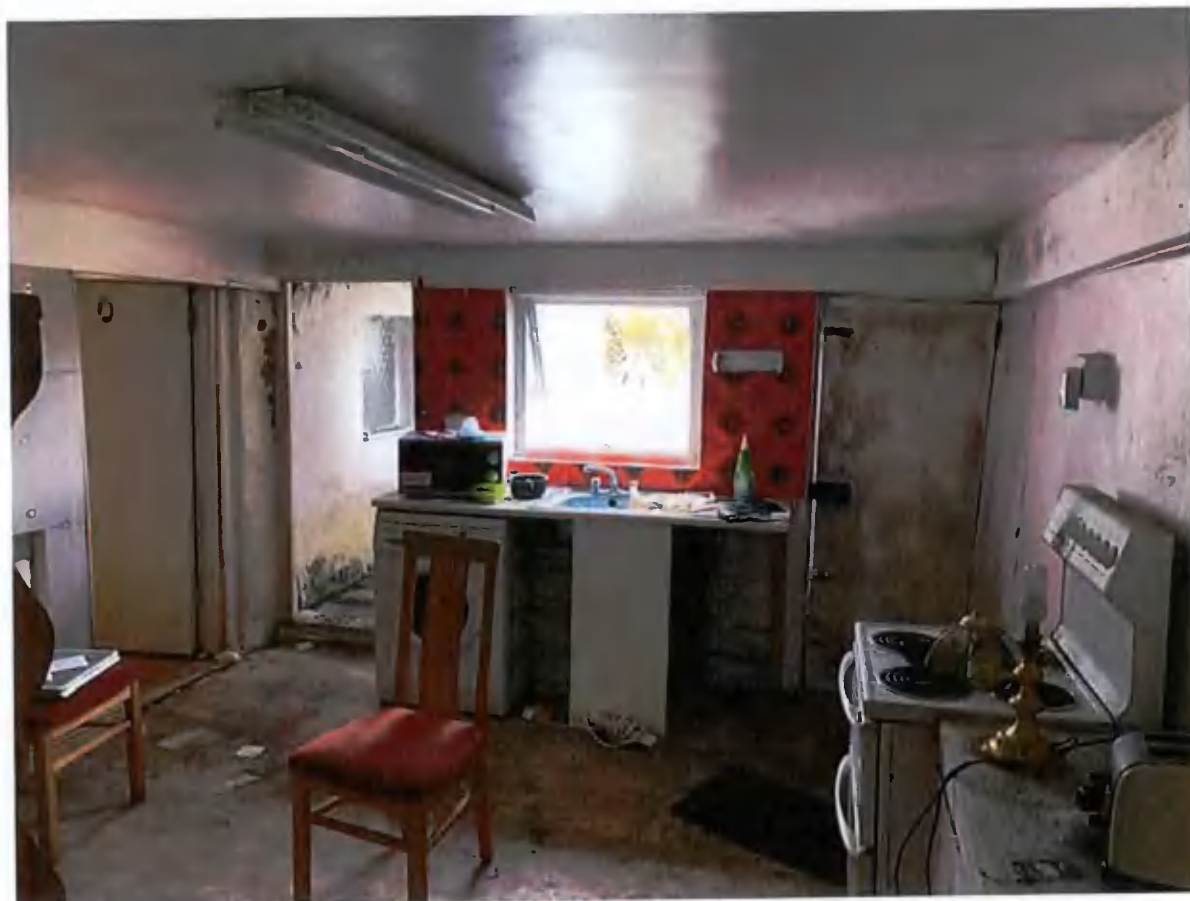
Figure 33 View of 20thC Kitchen Extension to north wall door openings
