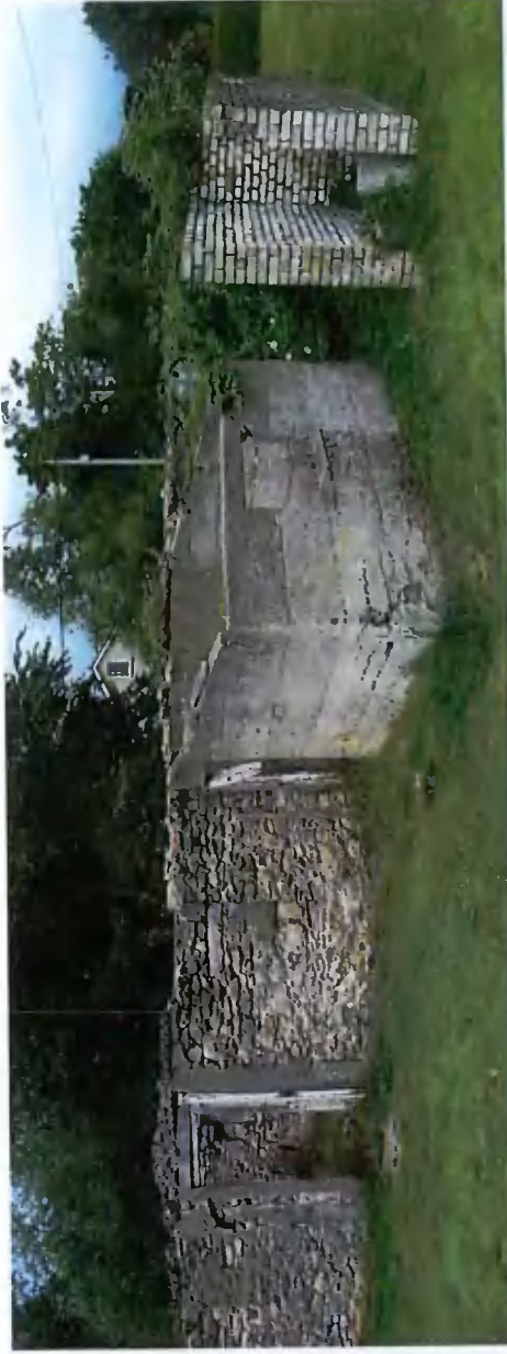
Fig. 52 – View of ruin walls along west boundary/ along Whitechurch Road, brick, concrete and rubble walling.
