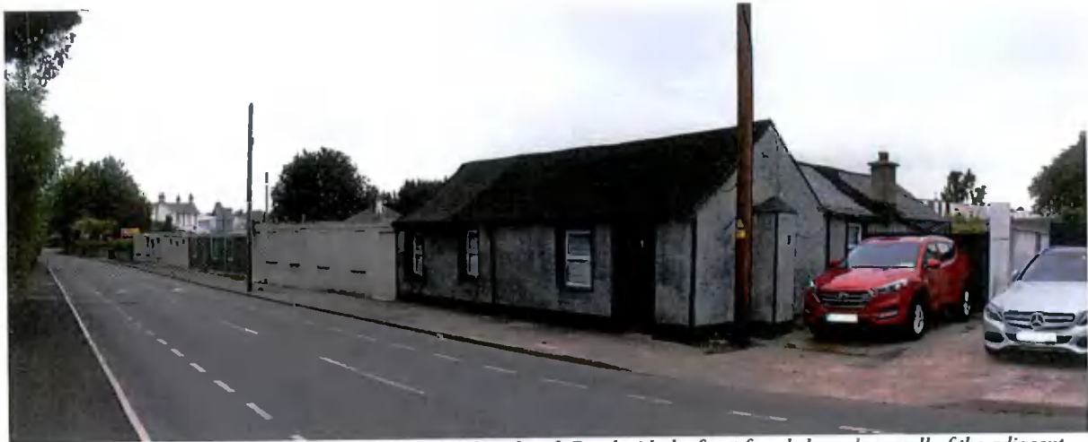
Figure 33 – The remaining cottage viewed from Whitechurch Road with the front façade boundary wall of the adjacent cottages along the pavement frontage of the site.
