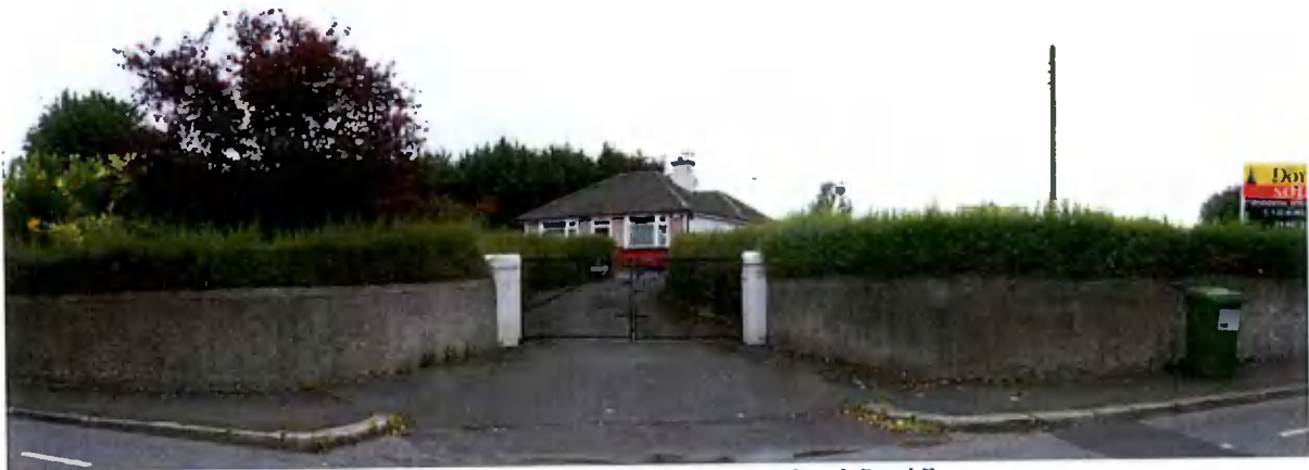
Figure 23 – Silveracre Bungalow from Whitechurch Road Entrance
