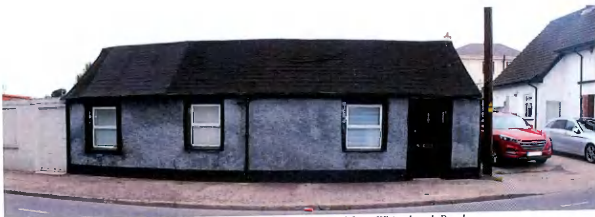
Figure 32 – The remaining cottage viewed from Whitechurch Road
