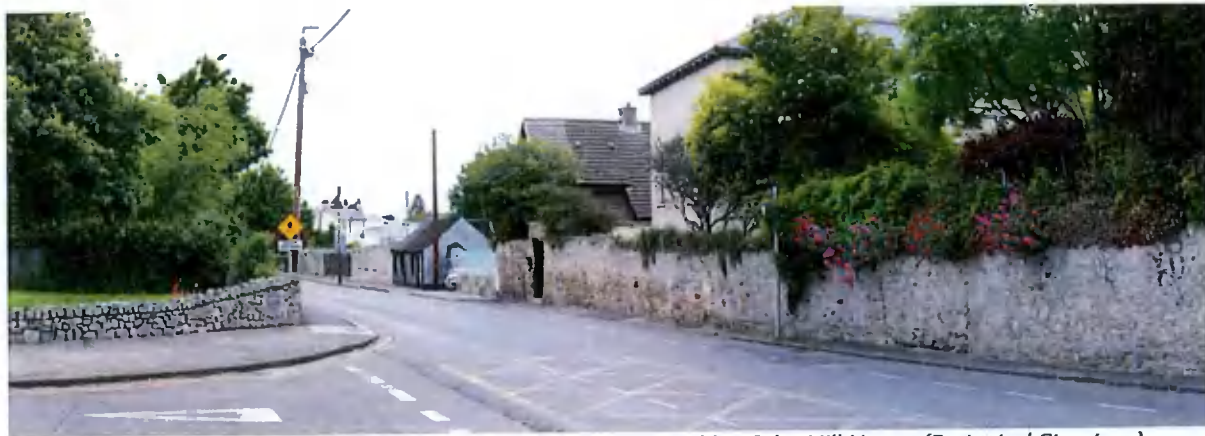
Fig. Existing view, Whitechurch Road view north along gable of the Mill House (Protected Structure)
