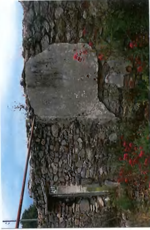
Fig. 52 – View of ruin walls along west boundary/ along Whitechurch Road, brick, concrete and rubble walling.
