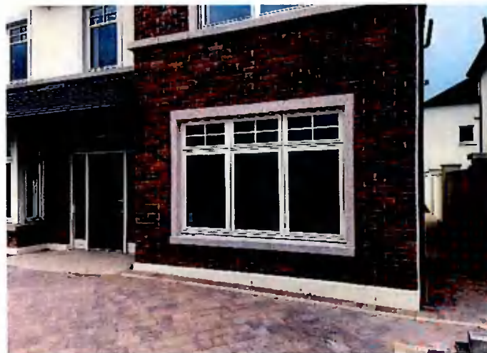
Fig. Material palette reference image of brick, granite and approach to detailing.
