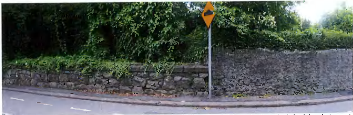
Fig. It is proposed to match the adjoining site boundary wall as illustrated above (wall on the left of the photograph)
