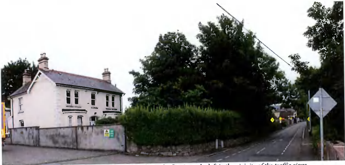
Figure 13: View south on Whitechurch Road – Site is on the left in the vicinity of the traffic signs
