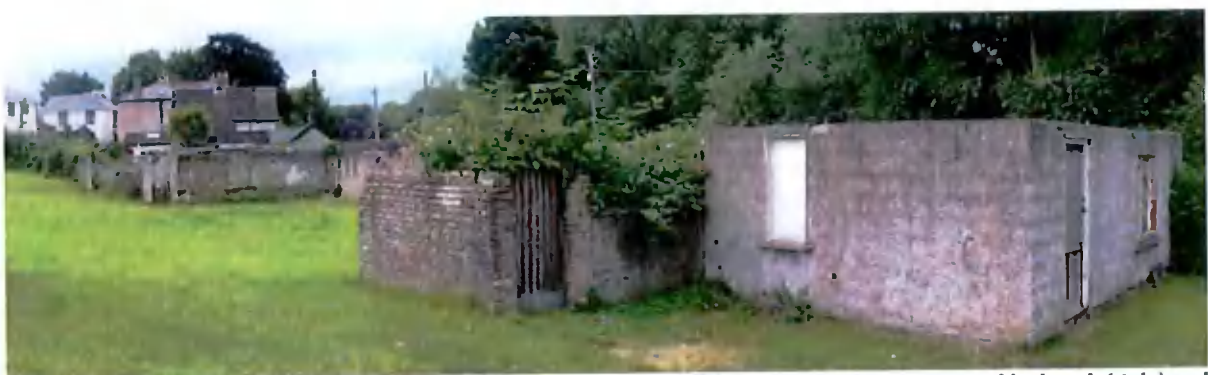
Figure 42 – The rear wall boundary wall of the first northerly cottage with ruined 20thC extensions in blockwork (right) and brick (centre) the houses in the background are on the site of the mill.
