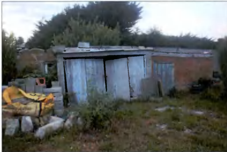
Plate 2 Building with Low Bat Roosting Potential.
