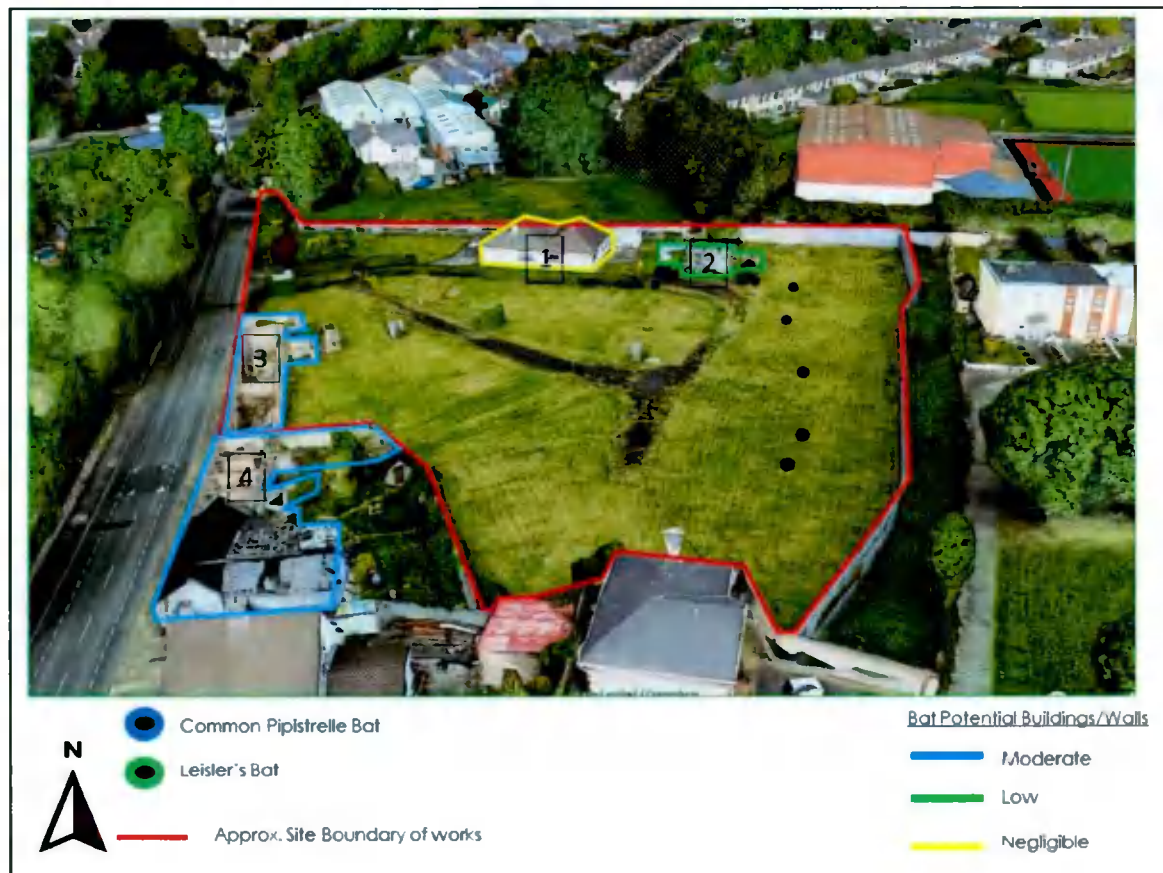
Figure 3 Buildings/structures onsite (labelled) with Bat Activity Map
