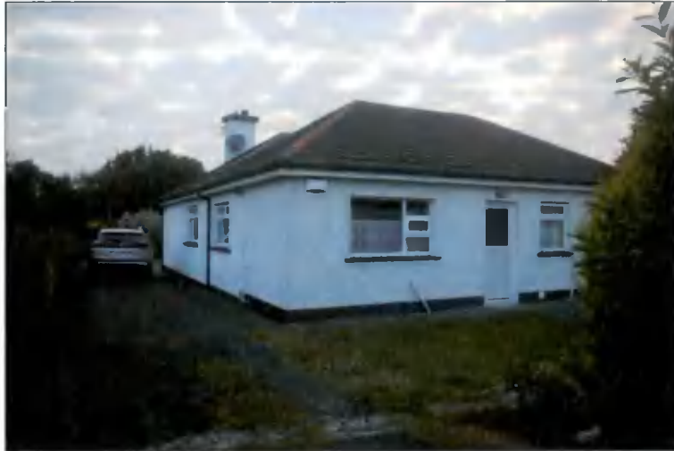
Plate 1 Main Building, currently occupied house, with Negligible Bat Roosting Potential.
