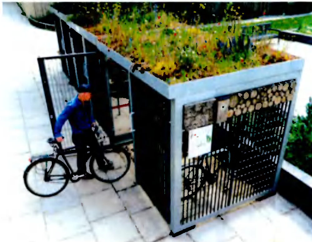
Figure 12: Example of sedum roof over communal bicycle parking building
