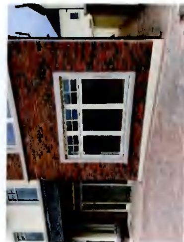
Proposed Wicklow Granite Window Reveals
