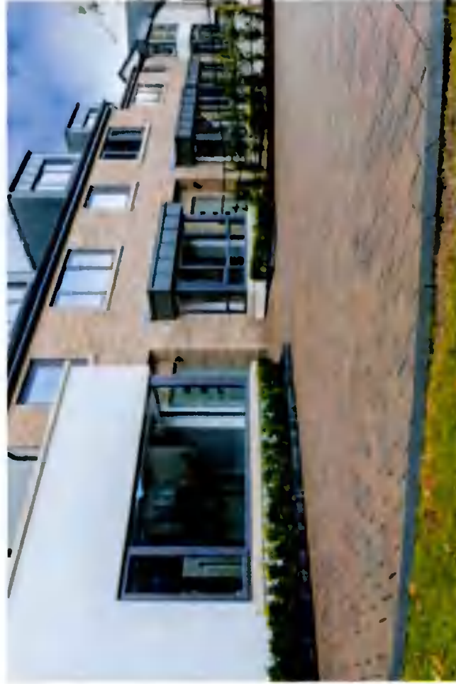
Fig 24. Example of permeable paving
