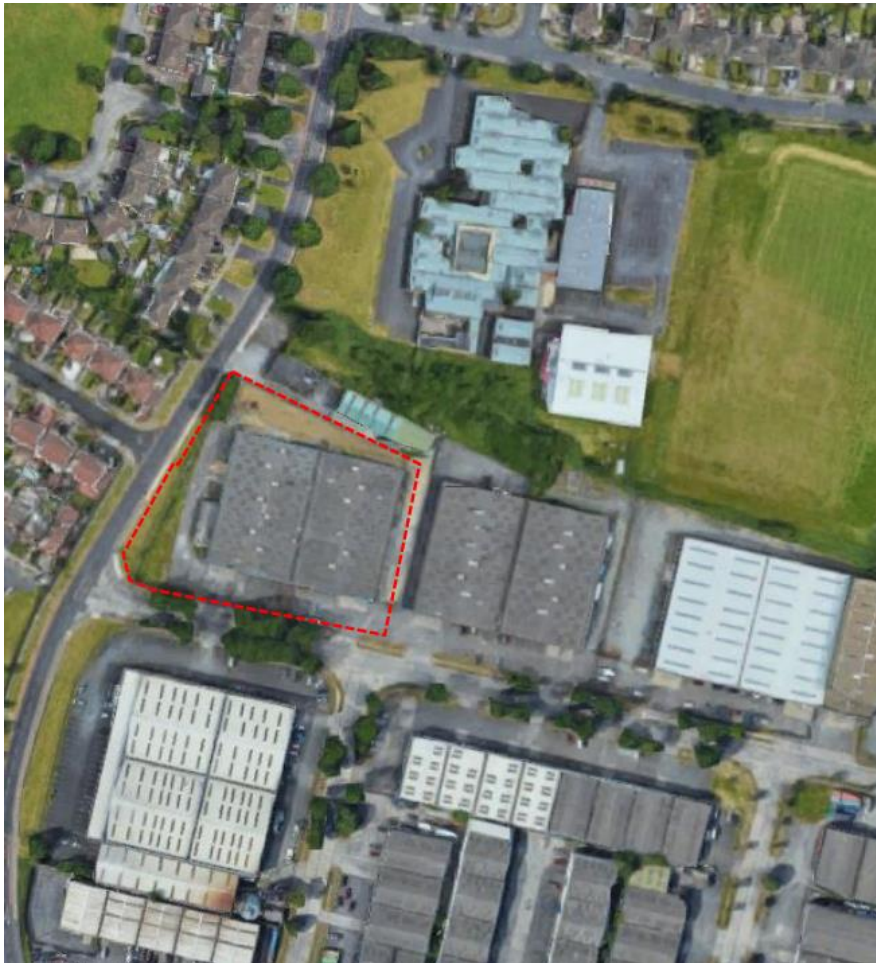
This image shows how close the ground floor school is to the building site
