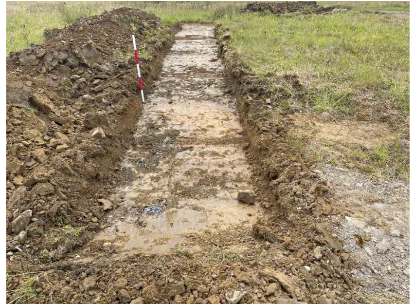
Plate 14: Test Trench 5, facing south.
