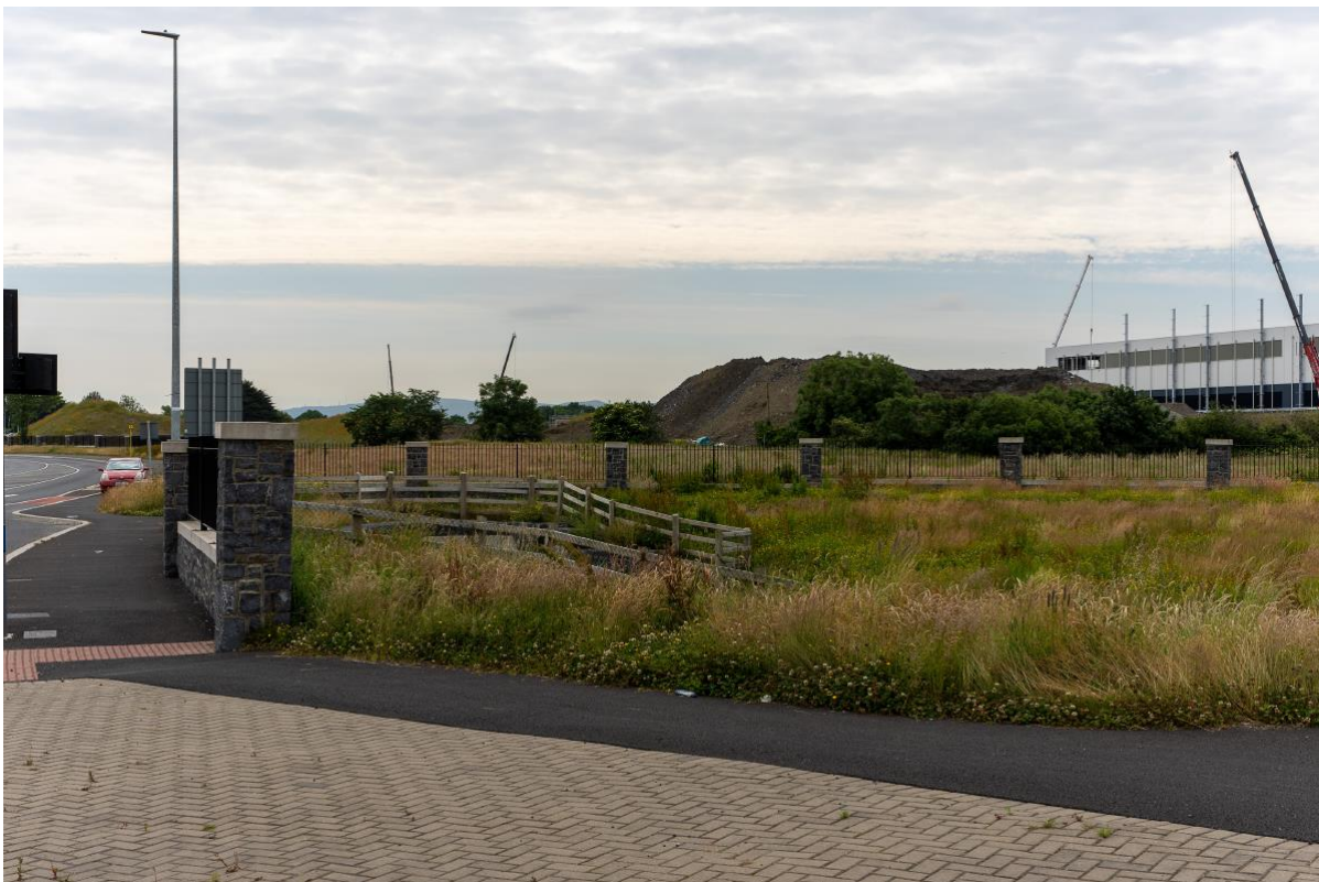
Figure 8-5: Viewpoint 2 - New Nangor Road at the roundabout junction with Baldonnel Road looking south east.
