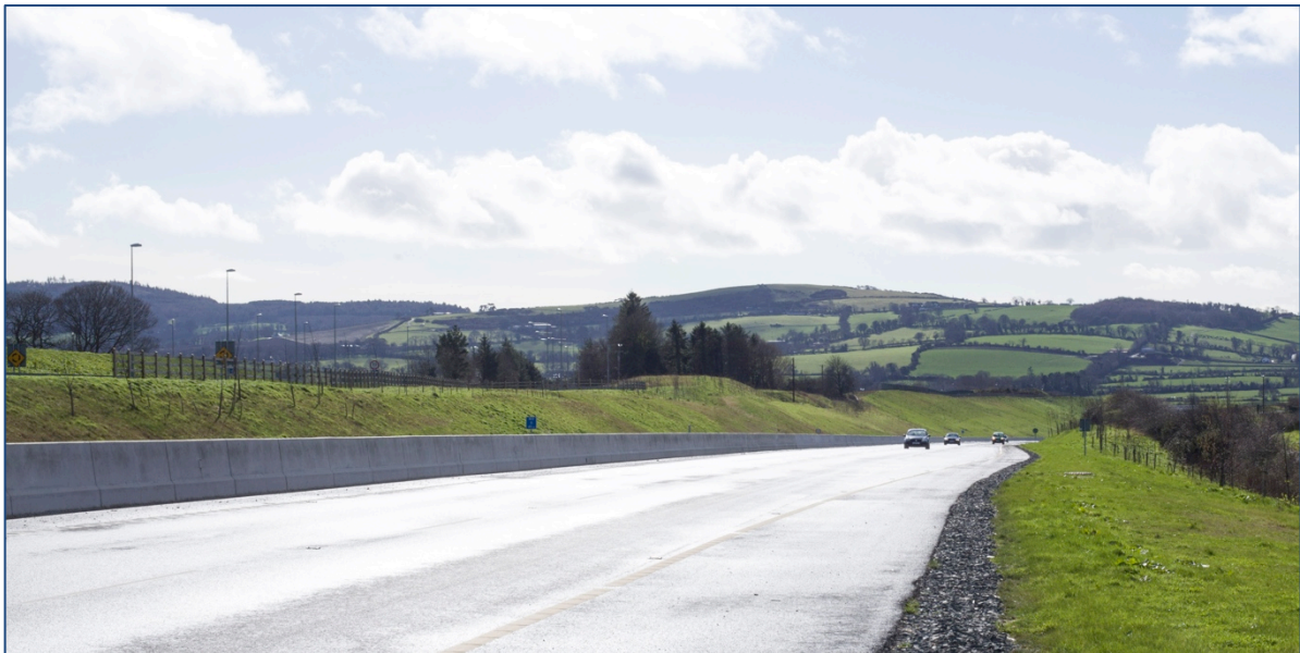
Figure 5: Similar levels of reflectance (to photovoltaic panels) emanating from wet road surfaces.
