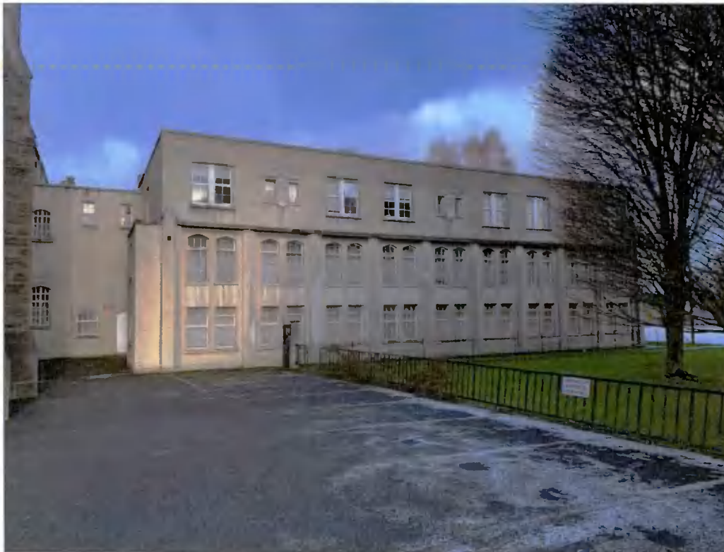
Plate 4: View of the library block built c. 1958
