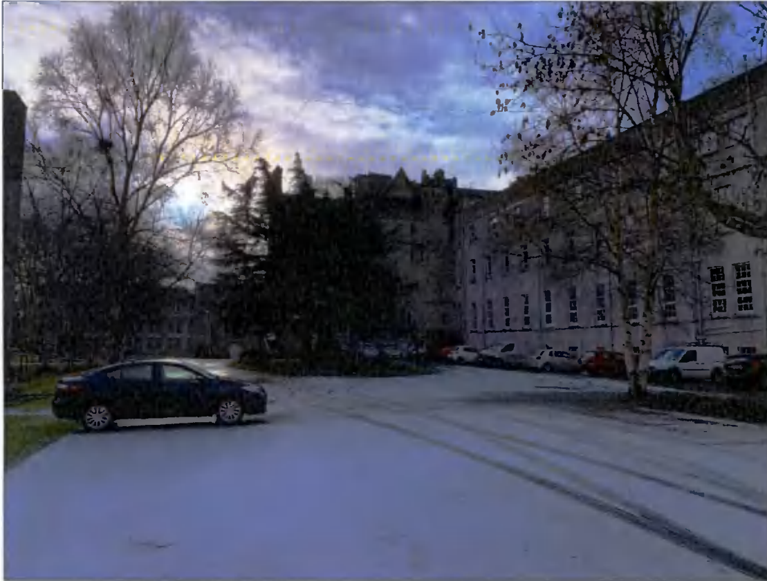
Plate 7: The late medieval tower is very much shielded from view due to its location at the “back of house” of the Priory and localised tree planting.
