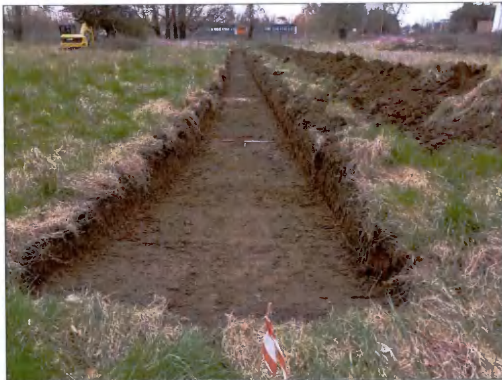
Plate 4: Trench 3 facing north
