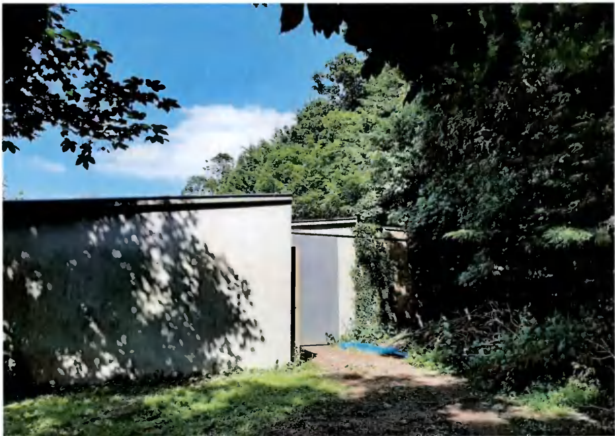
Figure 8.0 The rear of the existing stables structure, viewed from the South-West.
