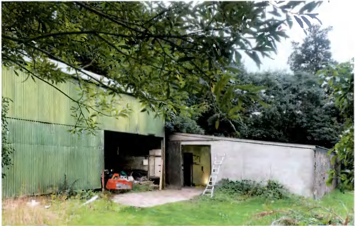
Figure 7.0 The front of the existing stables structure (right) and adjacent barn structure (left) viewed from the North.
