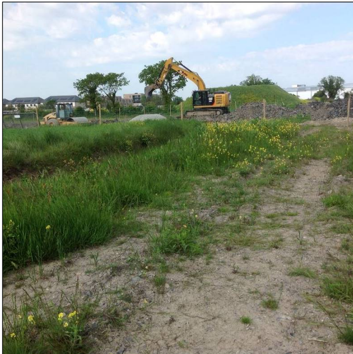
Plate 10. Celbridge link road – fenced wayleave in June 2021.
