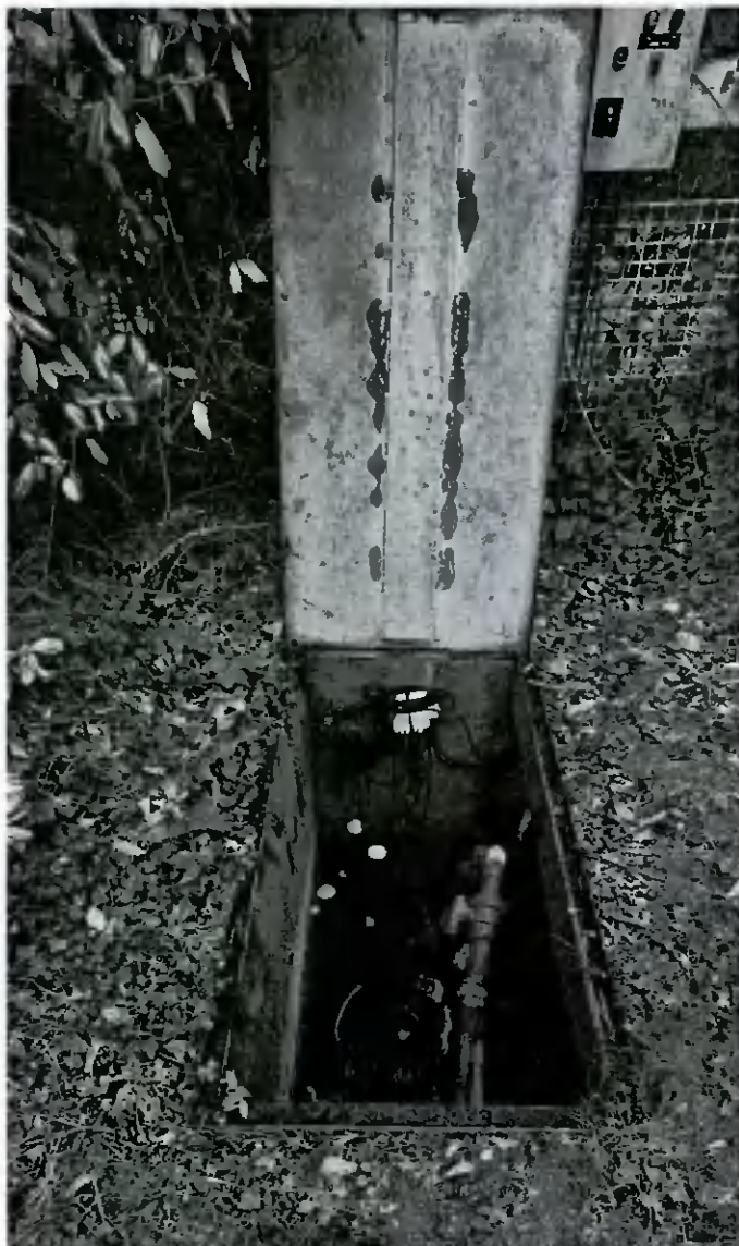
Fig 6. Existing pump chamber access manhole
