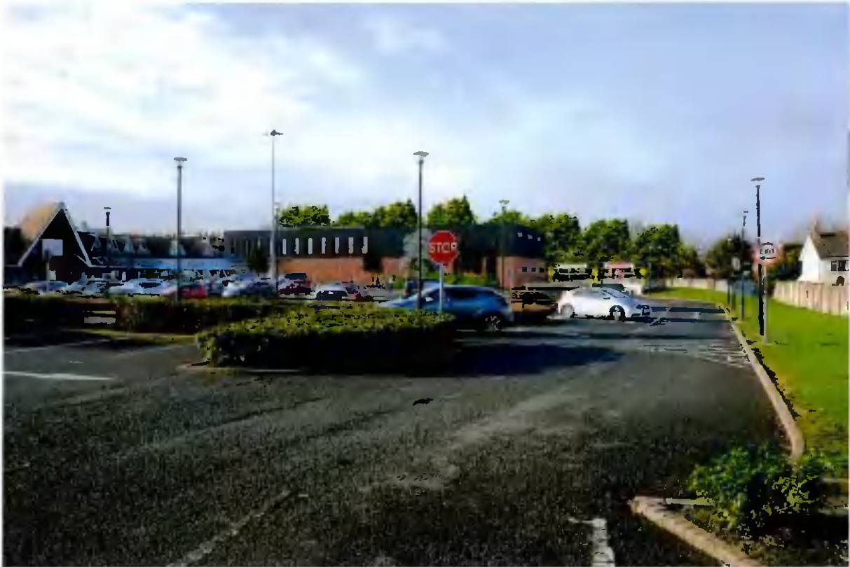
Photomontage of the proposed development, indicating amended signage, amended new canopy, amended fenestration, scale of development complements the existing shopping centre and surrounding areas.
