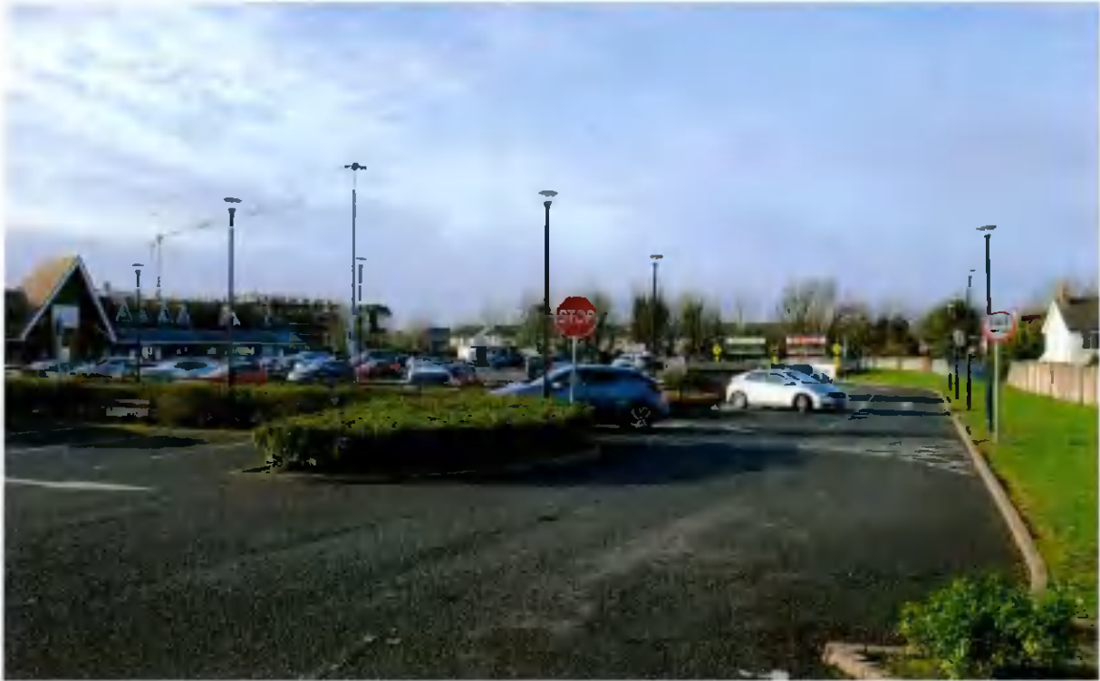
A large new residential development 'Somerton' is under construction, including a new multistorey apartment building directly adjacent, which can be seen with scaffolding surrounding to the rear of Lucan Shopping Centre, view looking West, January 2022.
