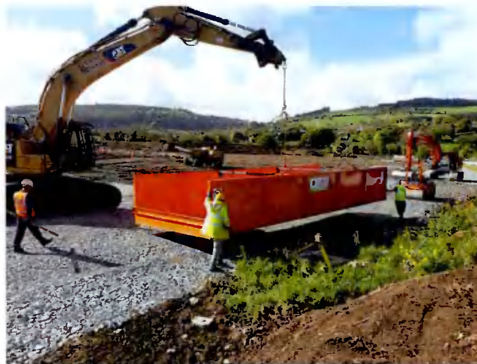
Fig 1 – Wheel being set up on site.
