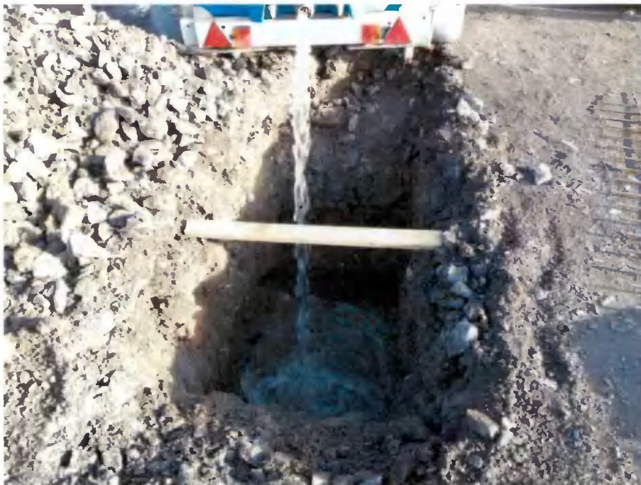
Figure 4. Filling ST1 with water
