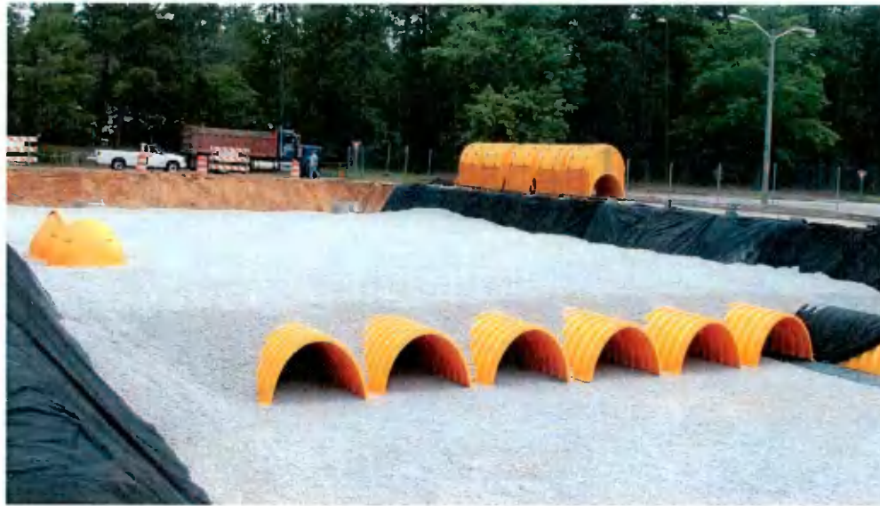
Figure 10 - Typical Cellular Storage (Stormtech) Installation
