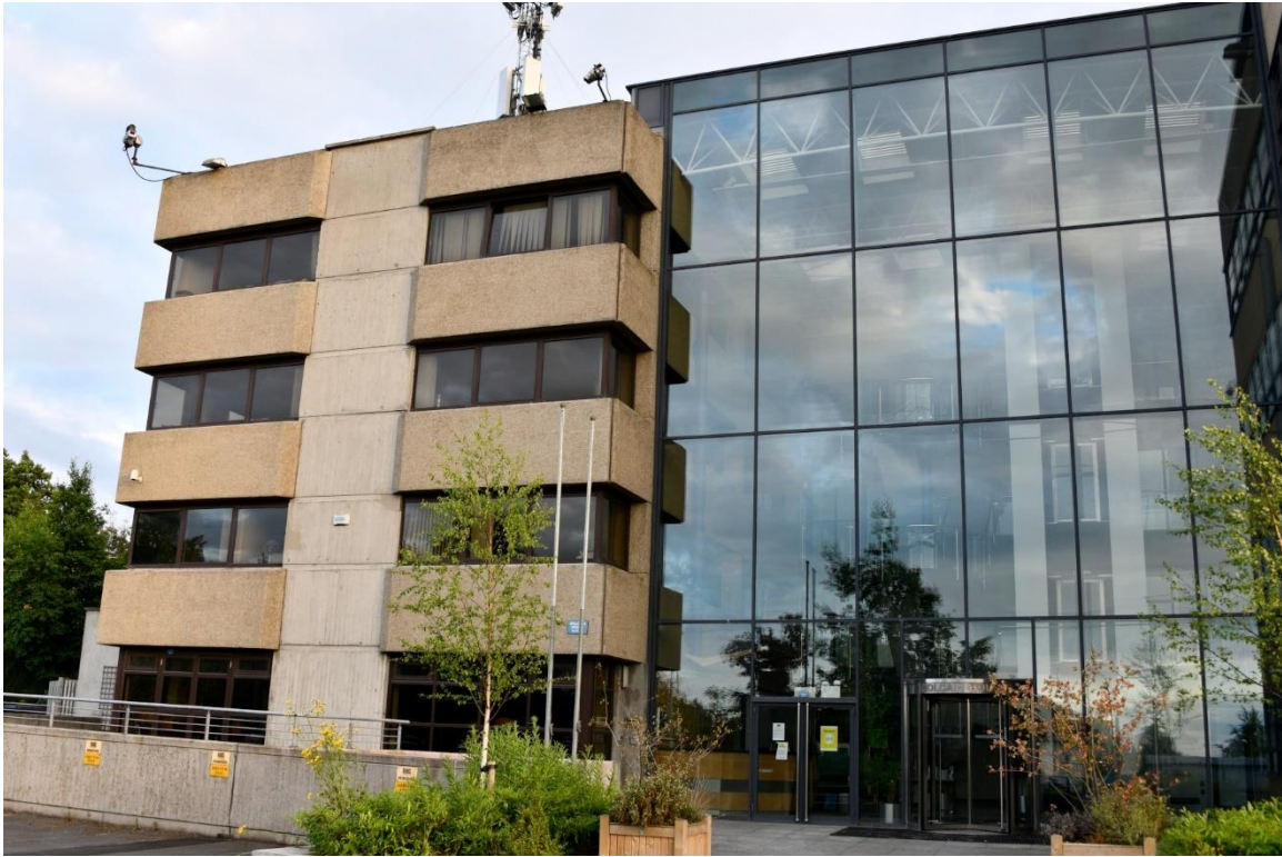
Plate 1: Buildings on site (Facing N).
