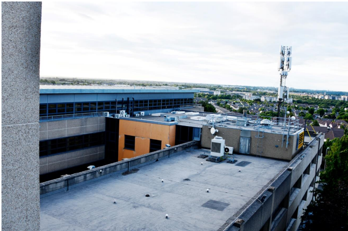
Plate 3. Exterior of Dolcain House.
