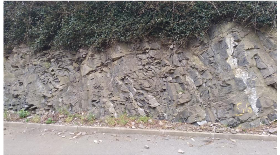
Plate 6: W side of the site showing excavated bedrock.
