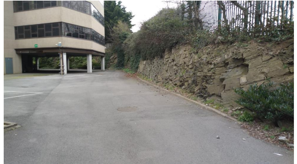
Plate 2: W side of the building, looking S
