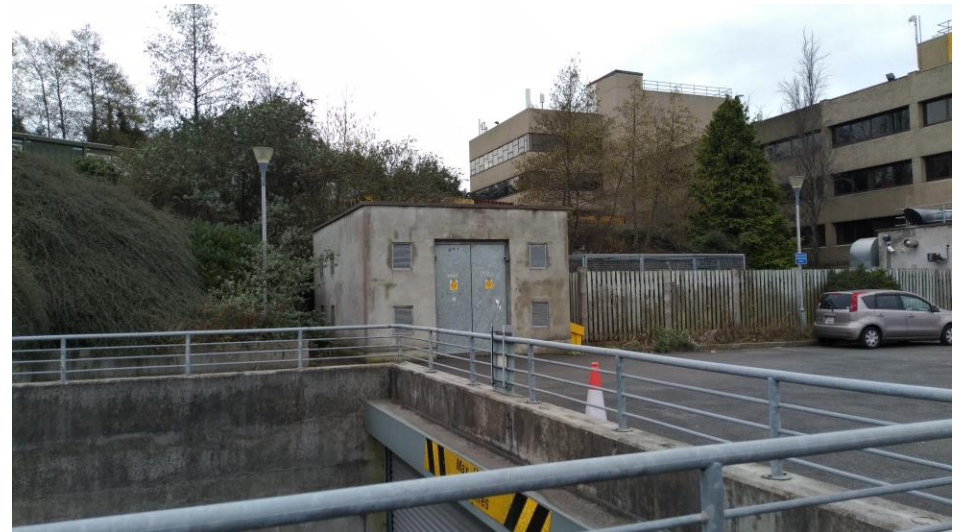
Plate 4: E part of the site with underground entrance visible, looking S
