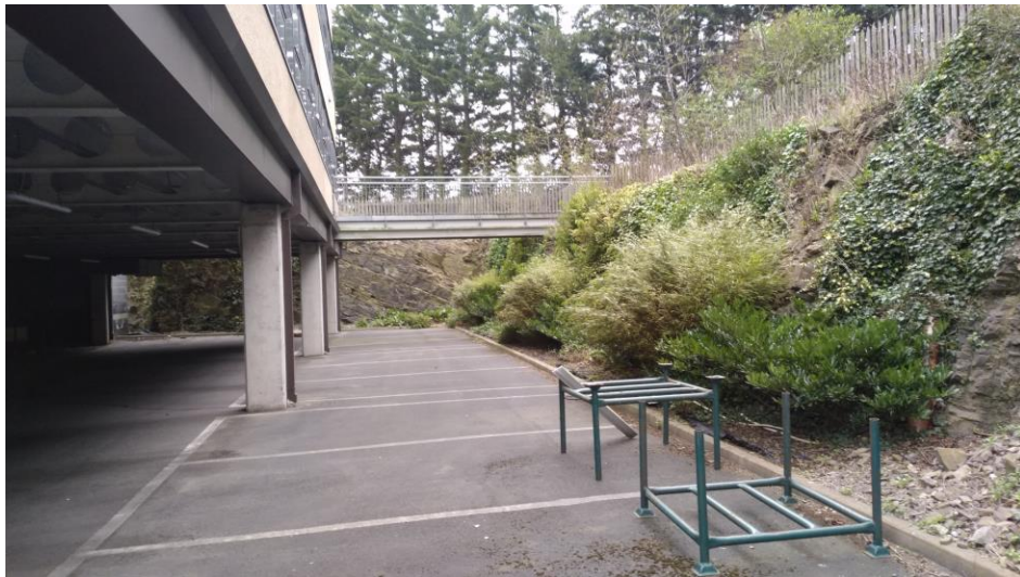
Plate 3: S side of the building, looking E
