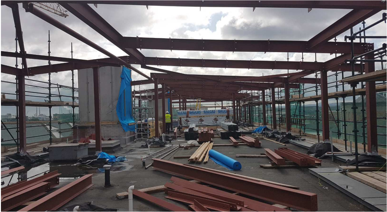
Figure 8: New floor built above existing as steel framed structure
