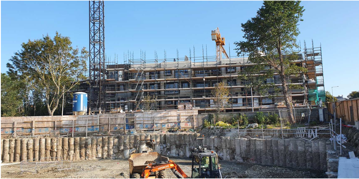
Figure 10 – New building under construction, perimeter scaffold in place for façade works
