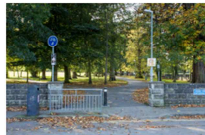
Shared Walkway/Cycleway at Bushy Park, Templeogue Road, Terenure
