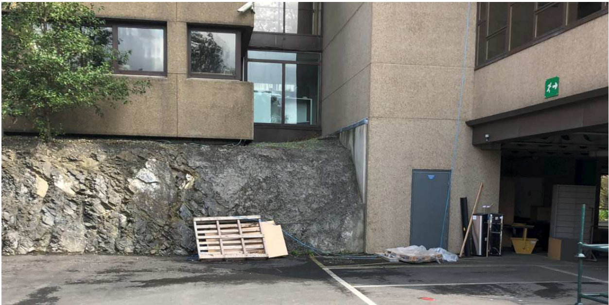
Figure 9: Site photo, west side of block B with bedrock from 1970s excavations visible. Several metres of rock have been removed in order to form the bitmac car park area in front. The floor of block B is bearing directly onto rock.
