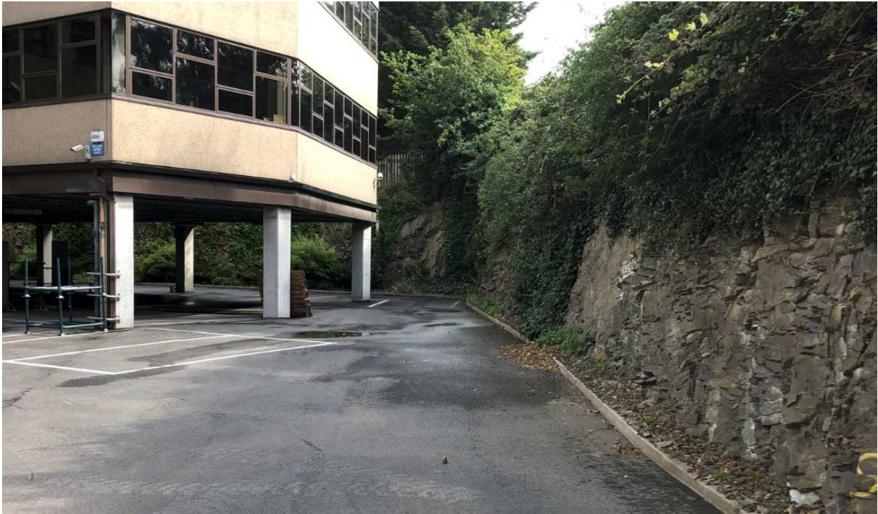
Figure 6: Site photo, west side of block C with bedrock from 2006 excavations visible and site boundary occurring at the pallisade fence visible at the top of the rock embankment (approx. 4.17m above bitmac level)
