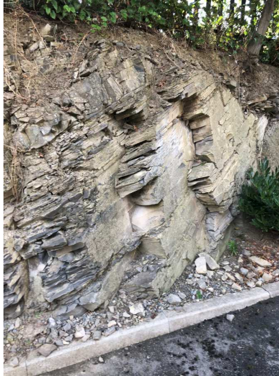
Figure 8: Site photo showing exposed rock face – existing bedrock is weathered limestone overlaid by 300mm of topsoil
