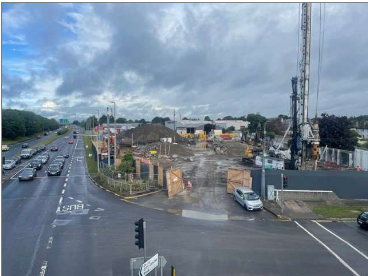
Fig. 1 – Palmerstown Strategic Housing Development Under Construction
