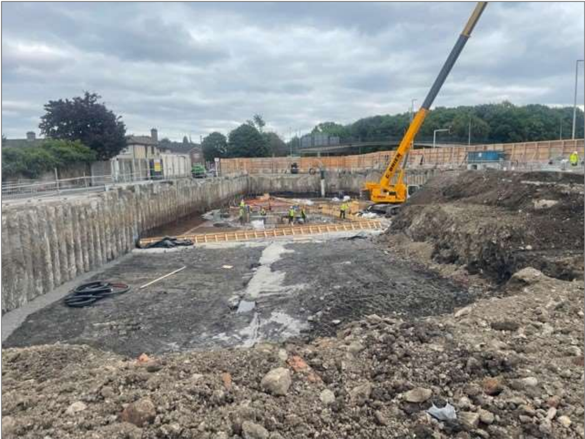
Fig. 2 – Palmerstown Strategic Housing Development Under Construction
