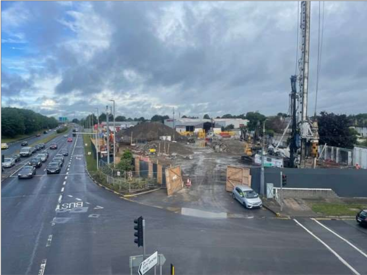
Fig. 2 – Palmerstown Strategic Housing Development Under Construction
