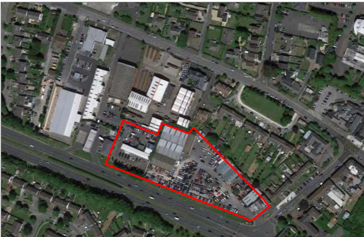
Fig. 1 – Aerial View (approximate boundaries of application site outlined in red)
