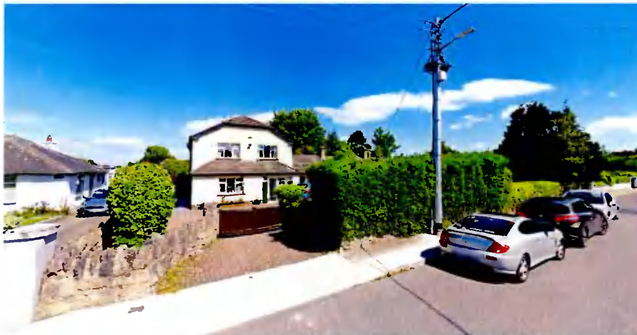
Two storey extension to the 10 Knockmeenagh Road – this dwelling has a much shorter setback to the street.
