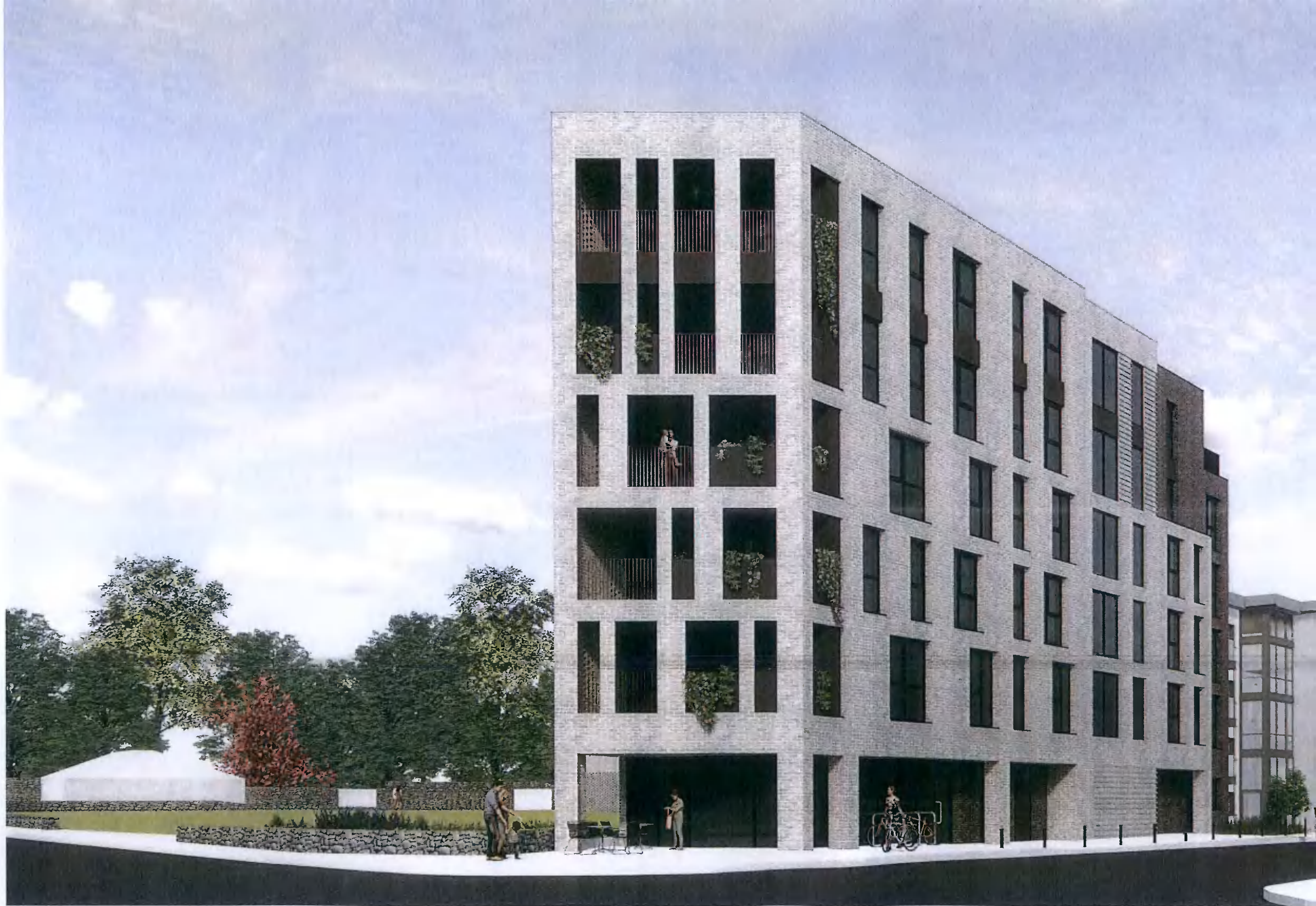
View from the Main Street / Greenhills Rd cross - BLOCK A south corner - Additional Information submission
