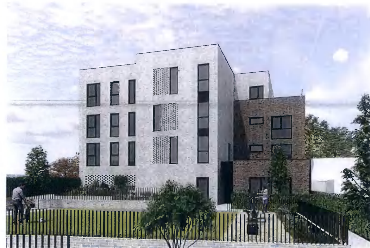
Rear facade of Block B (from internal courtyard) - Additional Information submission
