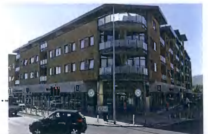
Priors Gate Apartment Building
