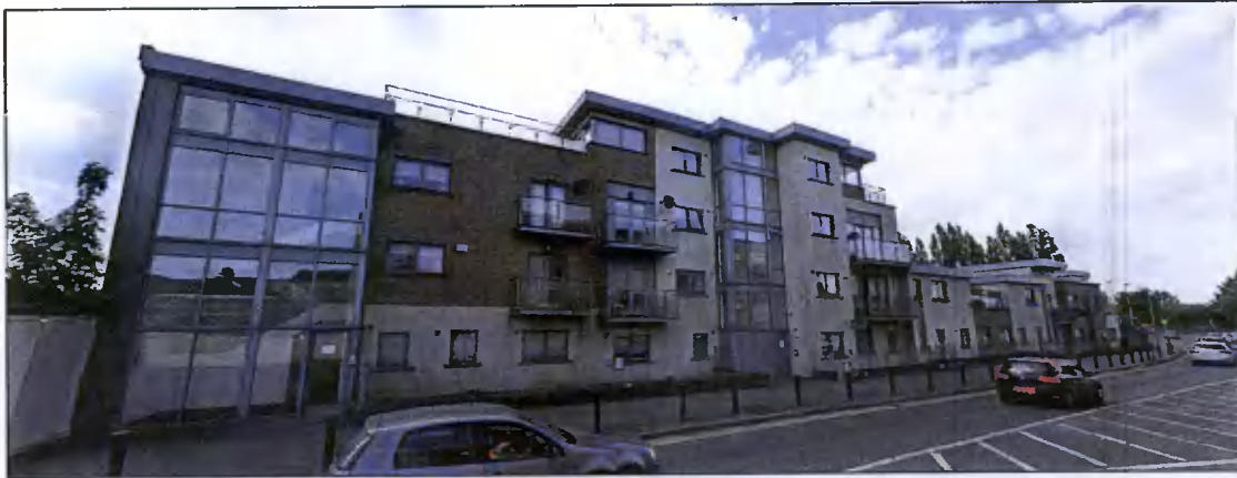
Figure 3. Street image of the existing Greenhills Court residential development (source: Google Maps, cropped by TPA, 2022).
