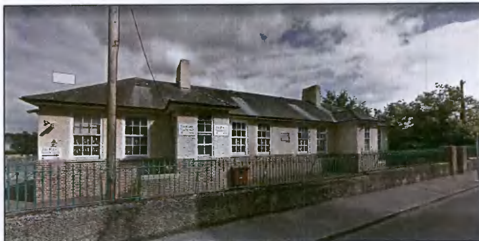
Figure 6. Street image of St. Basils Training Centre (source. Google Maps, cropped by TPA, 2022).
