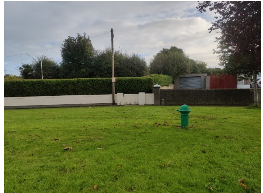
Plate 8: Location of the water pump NIAH Reg. No. 11213030, facing northeast.
