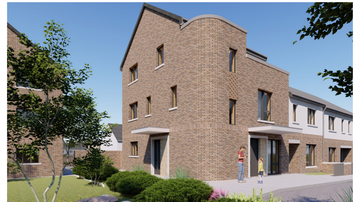
CGI of wide frontage units with landscape buffer and material change to signalise entrances
