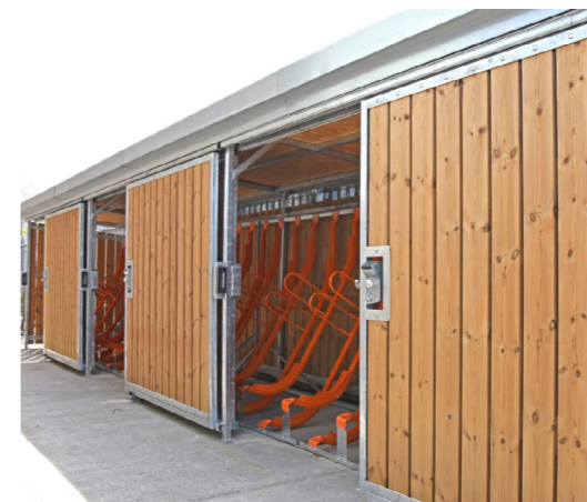
▲ Ref Image; Exterior of Enclosed Bike shelter with timber cladding & dual stacked bike racks
