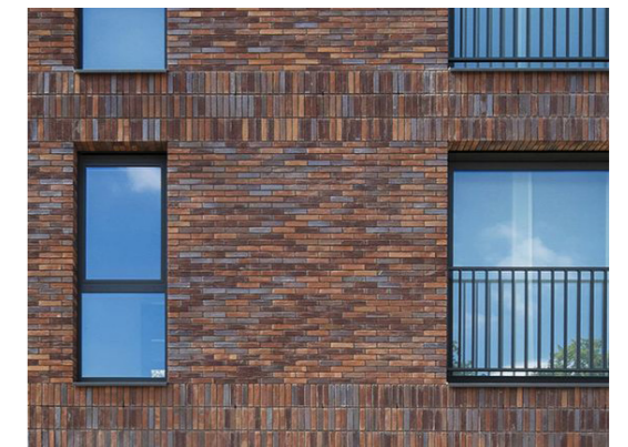
▶ Precedent image of brick facade with similar expression of brick banding & full height openings and contemporary fenestration
