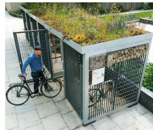
▲ Ref Image; Enclosed Bike shelter with steel structure & finish, and green roof to create a pleasing aesthetic
