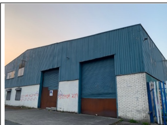
Photo 1: Building facing south
