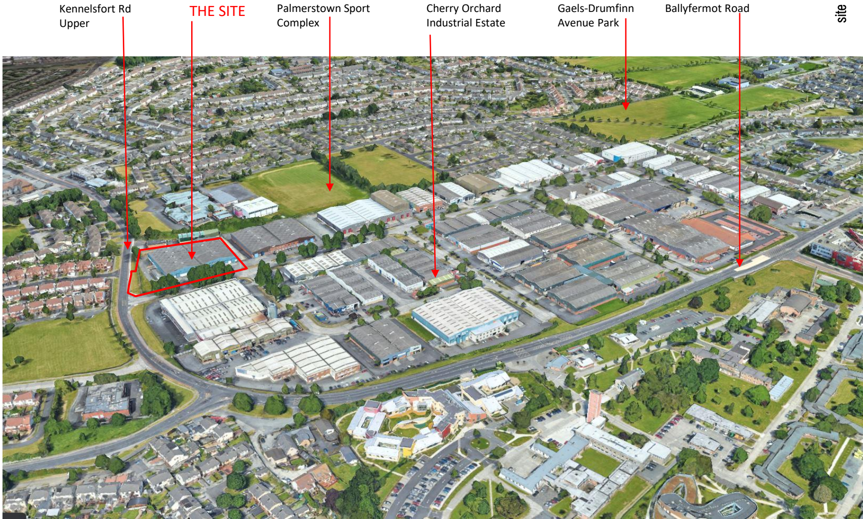
ORCHARD GATE SHD - Palmerstown Apartment Development
