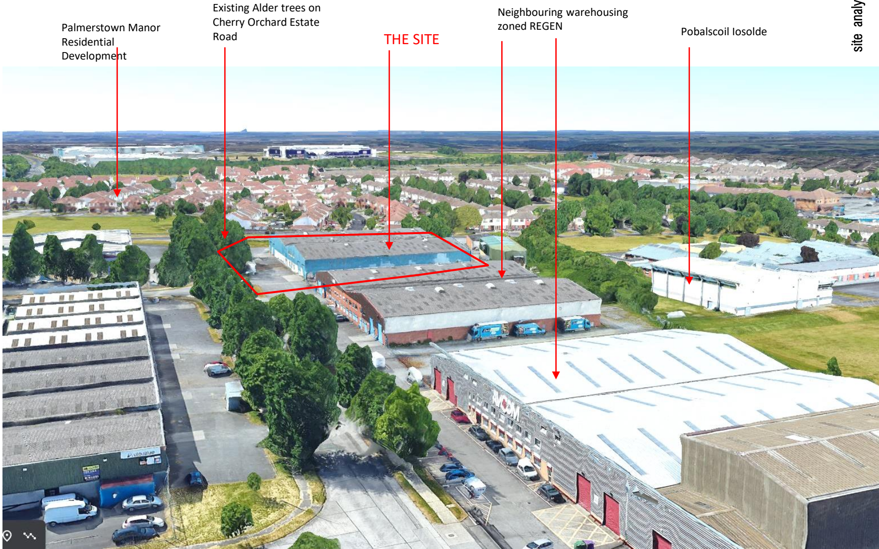
ORCHARD GATE SHD - Palmerstown Apartment Development
