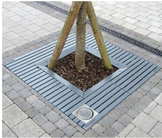
Galvanised metal grate flush with footpath allows surface water to permeate into the natural ground
