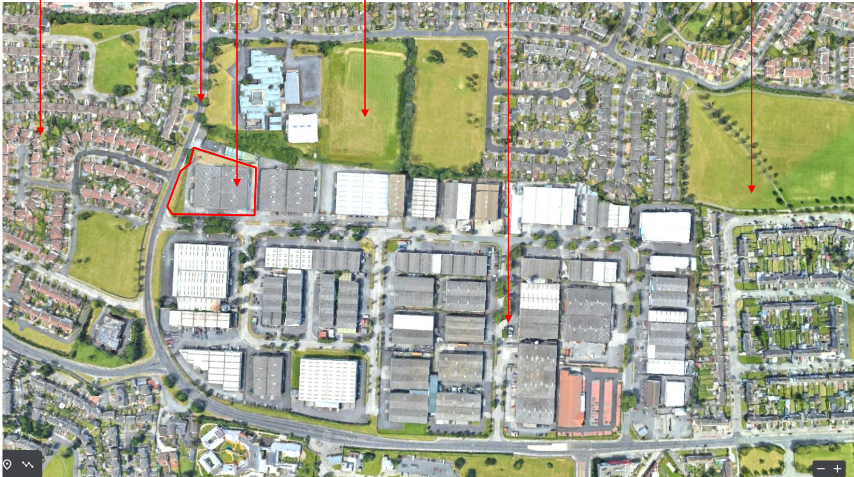
ORCHARD GATE SHD - Palmerstown Apartment Development
