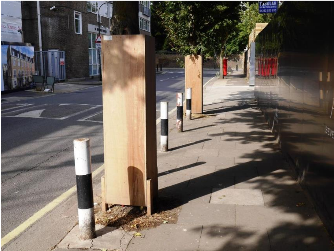
Photo 4: Example of timber stem protection to safeguard the stem of trees during construction works in close proximity.
