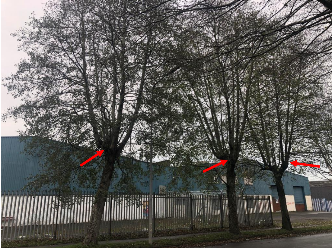
Photo 1: View of the Italian alders T290 to T292 located adjacent to the southern boundary. The red arrows indicate the points at which the trees were previously topped and have now produced multiple mature vertical branches that are considered to be weakly attached.
