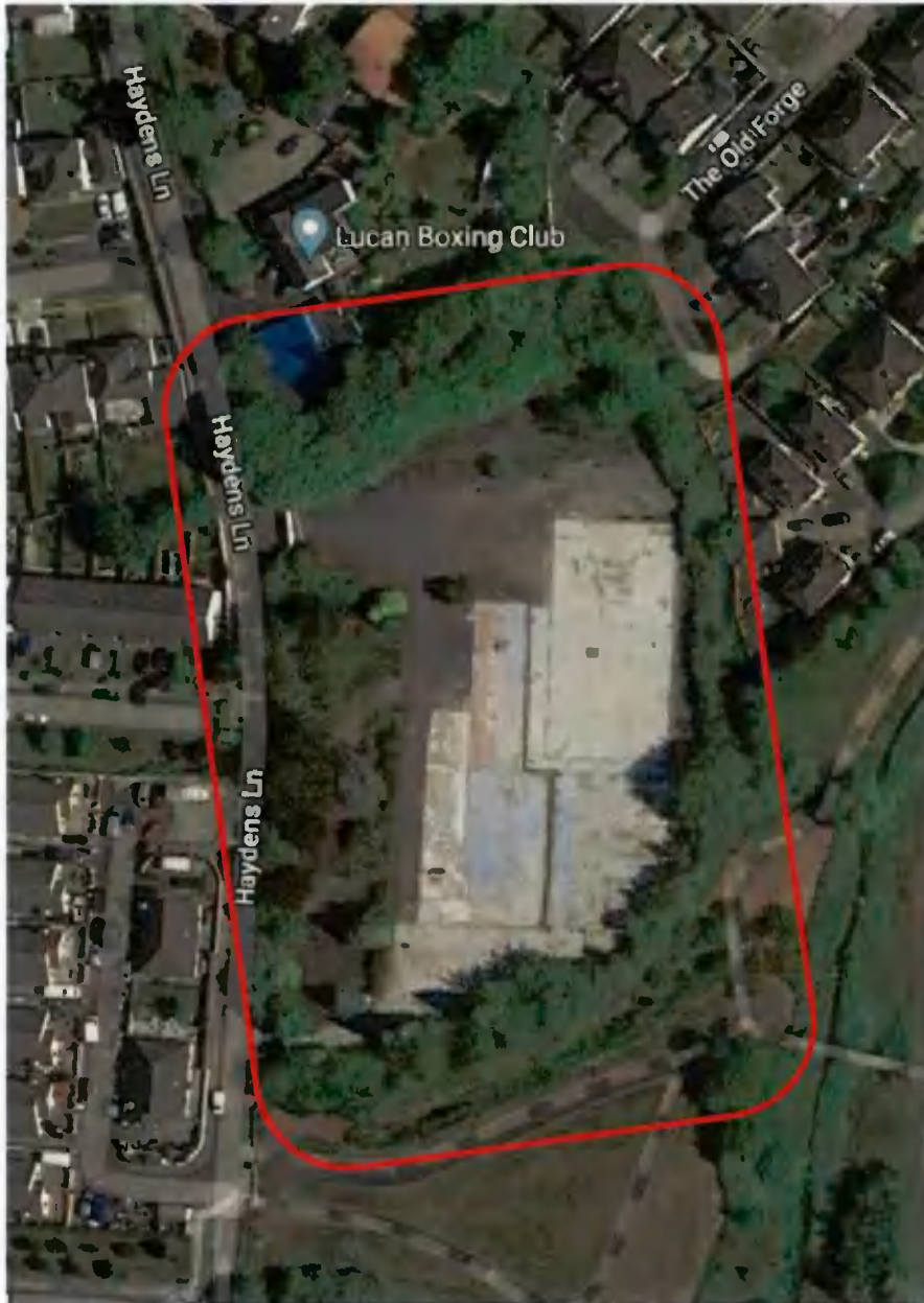
Figure 1a: Aerial photograph of proposed development site: Hayden's Lane, Lucan, Co. Dublin.
