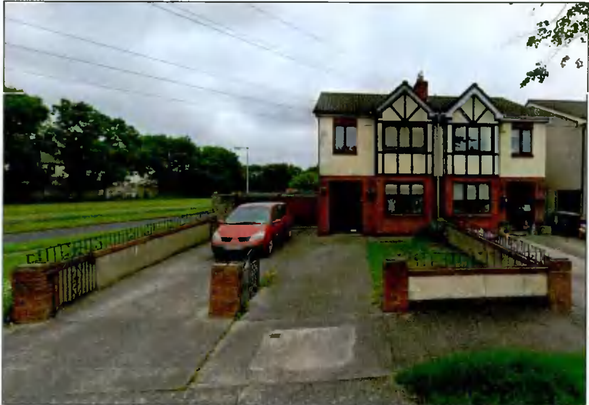
Plate 2.6: Google Streetview extract of site's frontage
