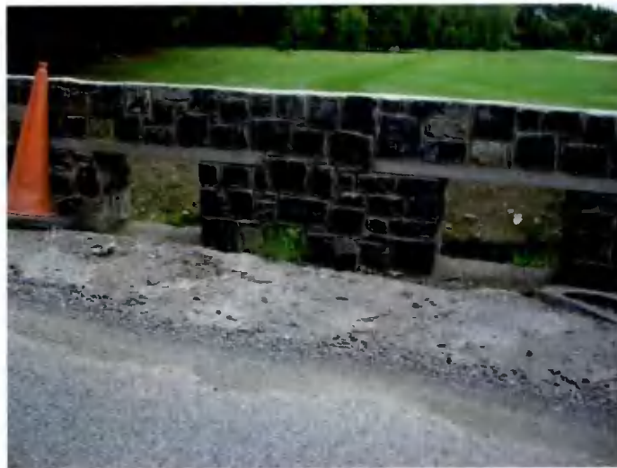
Figure A5 New Opes After Wall Reinstatement 2010
