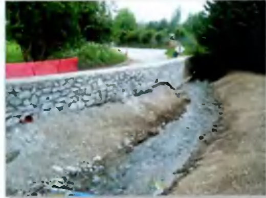
Figure A4 After Wall Reinstatement 2008
