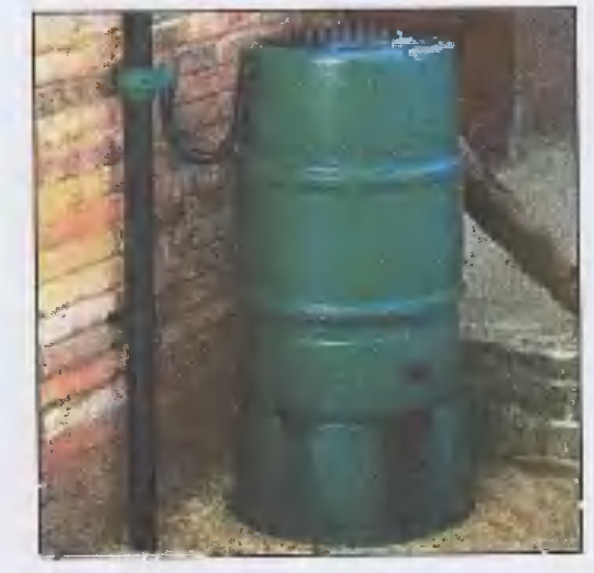
Typical 220 litre Rainwater Butt N.T.S.
