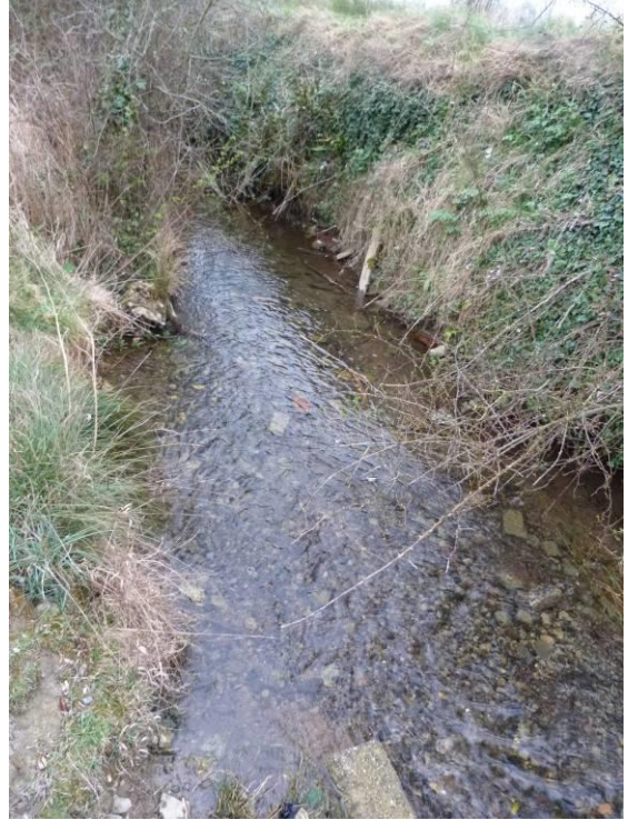
Plate 28. The drainage channel (overflow for the Canal) – this stream runs eastwards along the southern boundary of the site.
