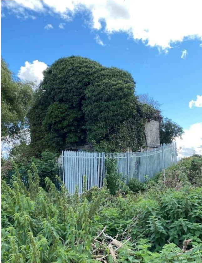
Plate 13.8 – Omer Lock House (RPS 122/NIAH 11205011), facing southeast
