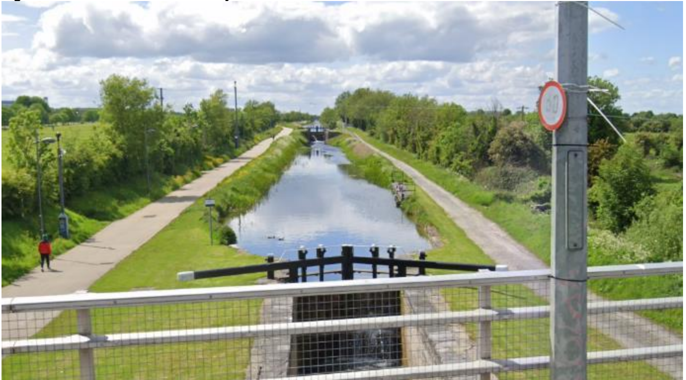
Figure 10.8 – Grand Canal Greenway from Fonthill Rd
