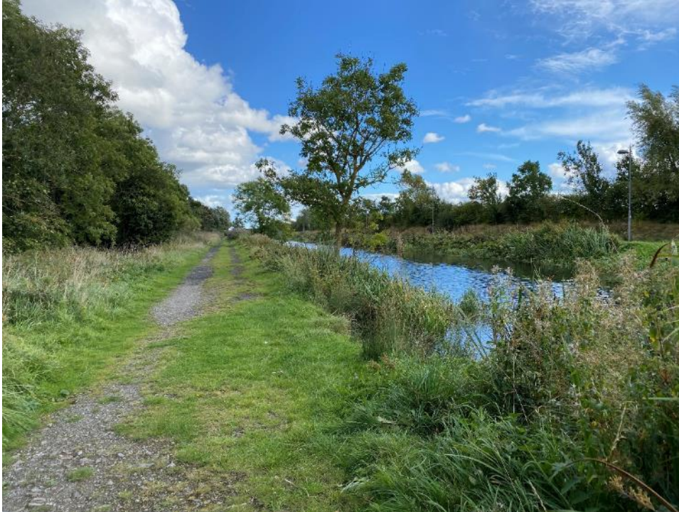
Plate 13.7 – Grand Canal, facing east
