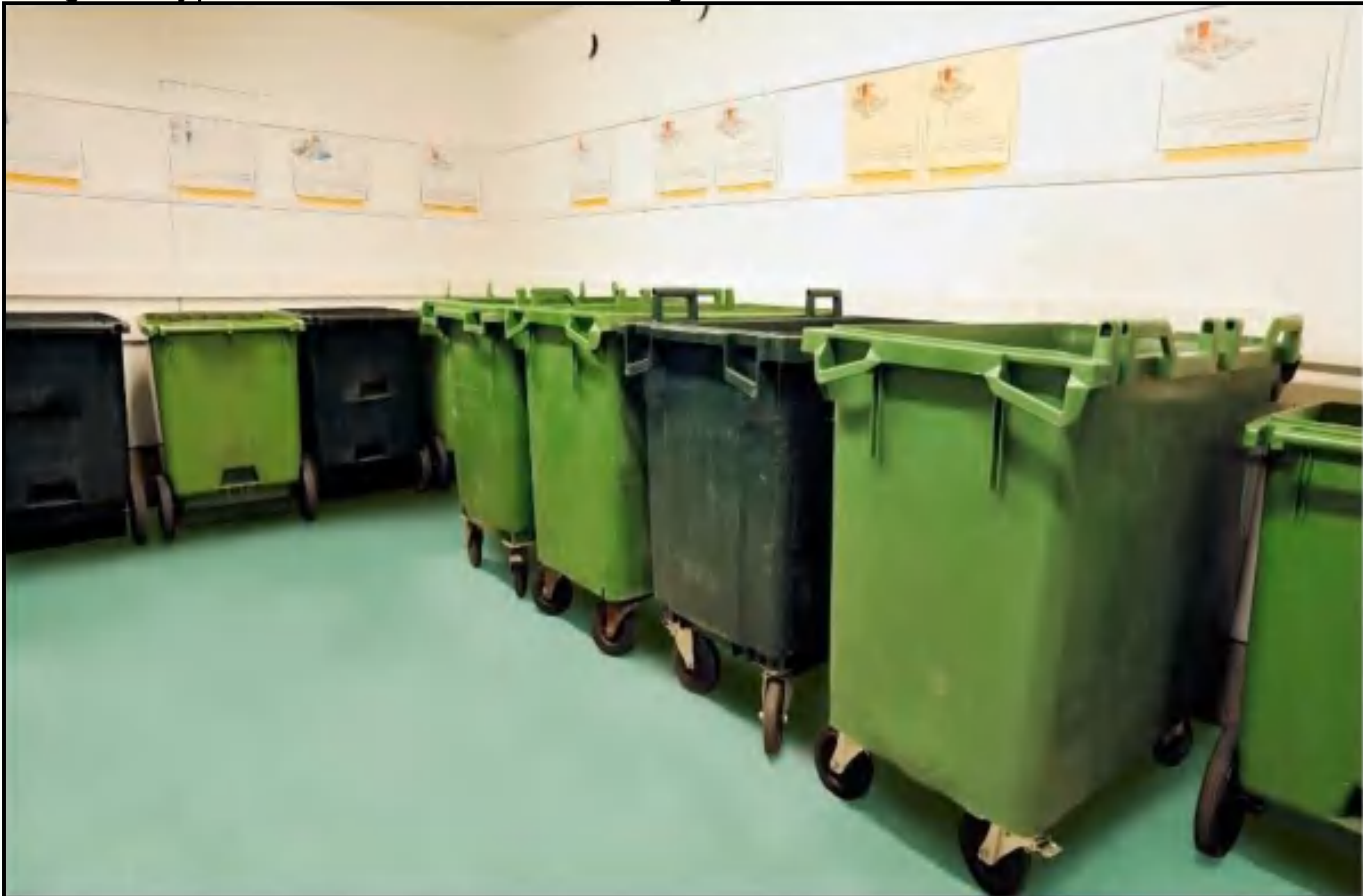
Image of Typical Communal waste storage area
