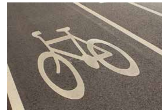
Asphalt Cycleways with Line Marking
