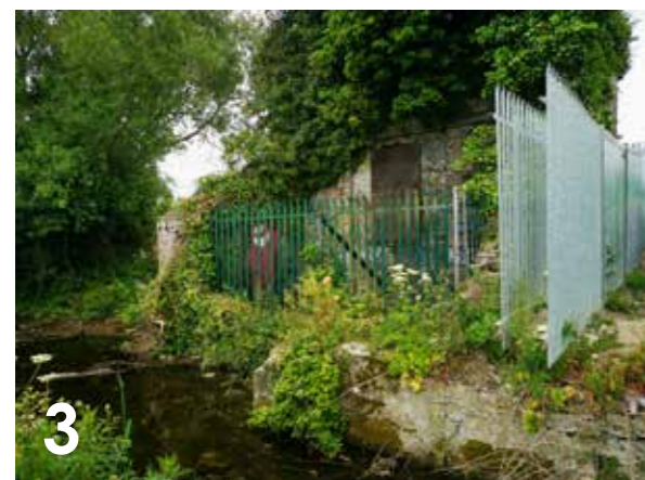
3 Overflow stream adjacent to Omer Lock House
