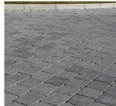
Concrete Block Paving to thresholds and private paths
