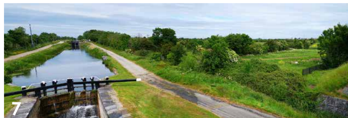
7 View from R113: Existing canal buffer vegetation adjacent to canal path
