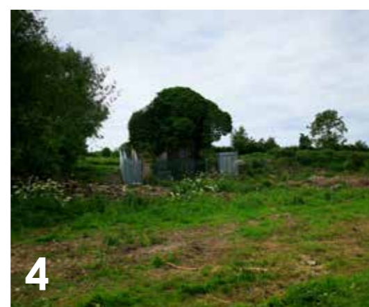
4 Omer Lock House - derelict & overgrown
