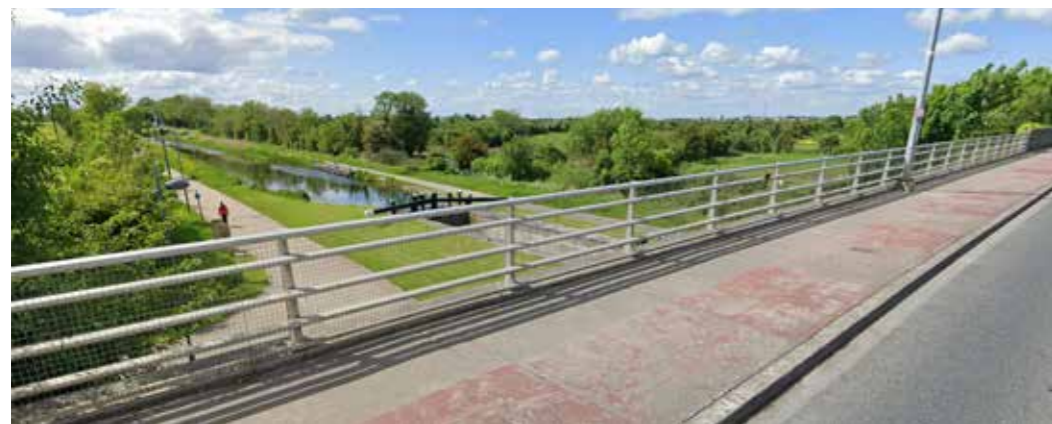
View north-west towards site from Grand Canal roadway crossing
