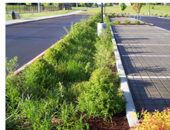
Planted Swales and permeable paving
