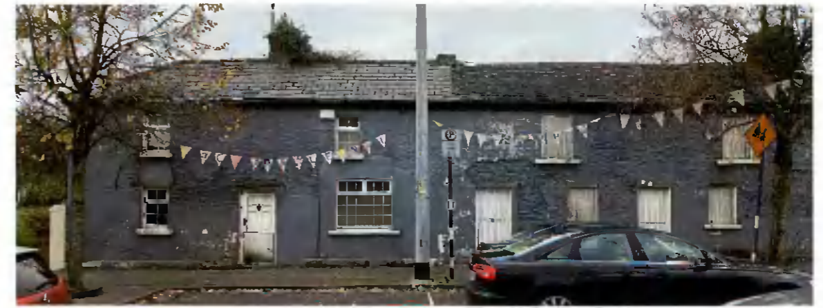
PHOTOGRAPH: FRONT ELEVATION
