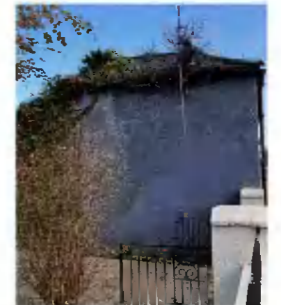
PHOTOGRAPH: END ELEVATION
