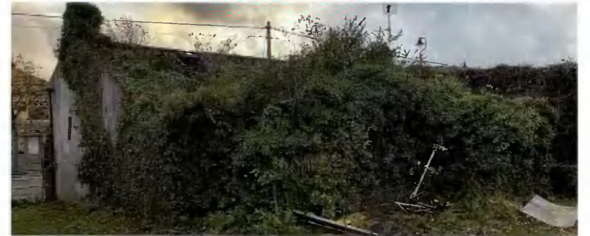
PHOTOGRAPH: REAR ELEVATION
